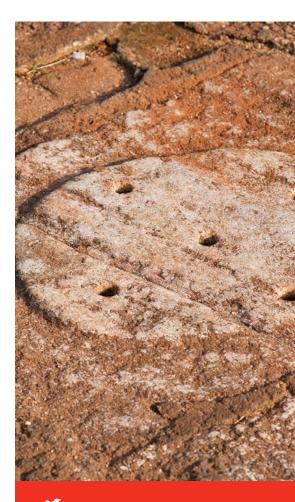
Relying on natural resources and simple physics, the water fountains in the rock fortress were powered by the accumulation of water from the top of the rock. Gaining momentum as it rushed down, enough pressure would be created to allow to the water to shoot through the holes creating a beautiful and relaxing sight at the varied water gardens.
