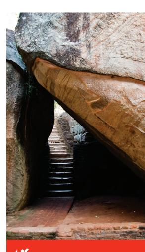
In order to prevent water from seeping into the cave, drip ledges have been cut into the rock, thereby protecting the interior. The cut away section has been decorated with art and has been created in a manner that protects even the artwork from the elements.
